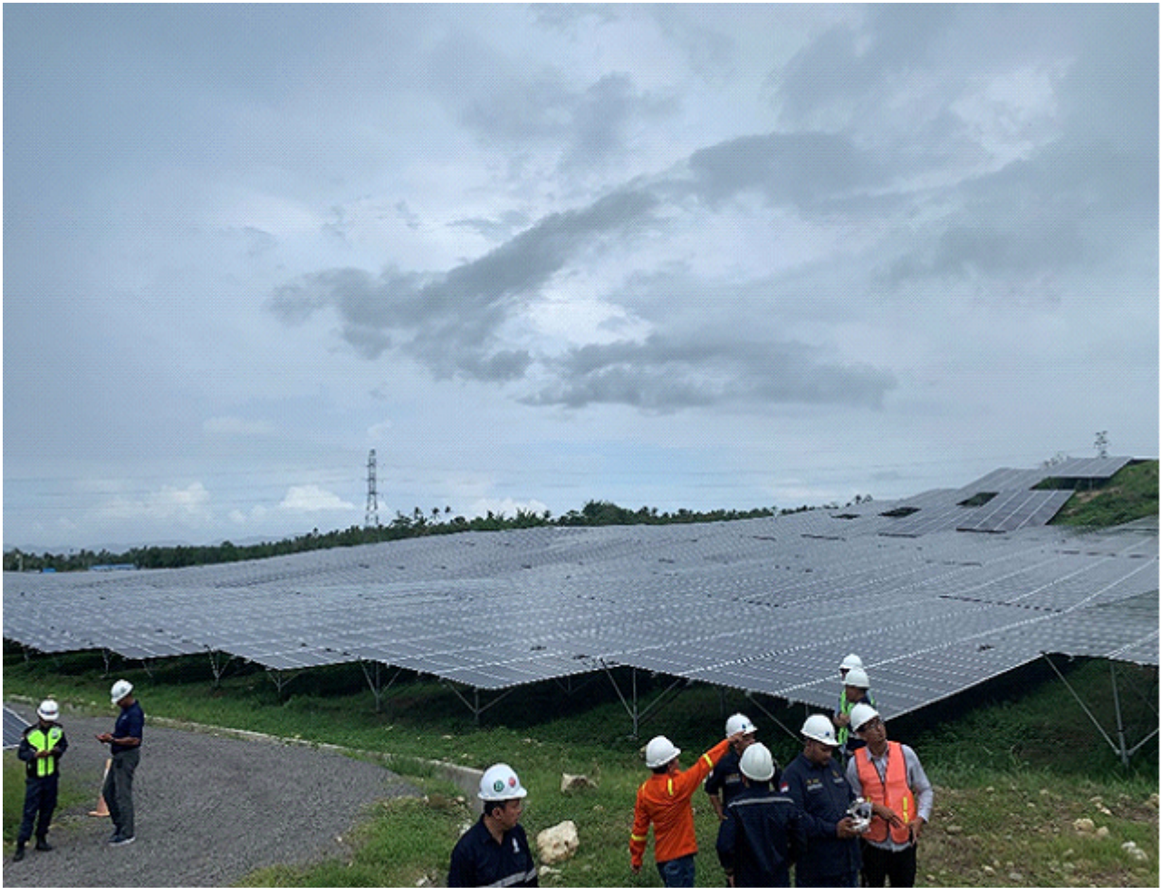
Figure 1. Site Visit to Solar Power Plant
